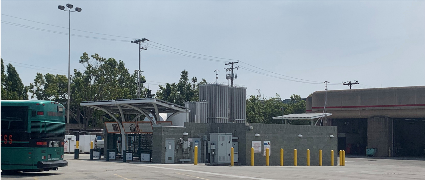
Figure 2. Hydrogen fueling yard at AC Transit, an Oakland, CA based public transit agency
