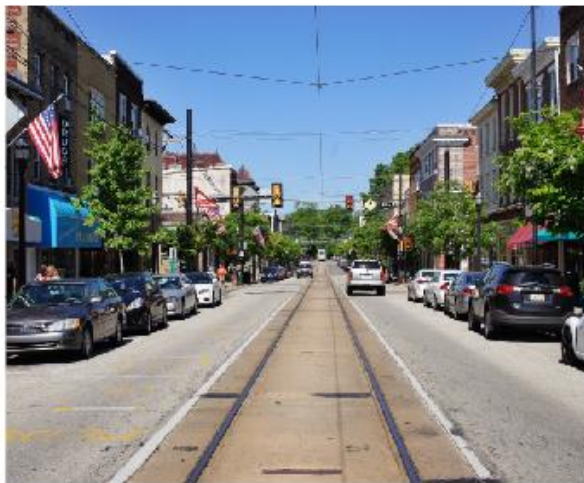
Existing Conditions on State Street: Single-track
