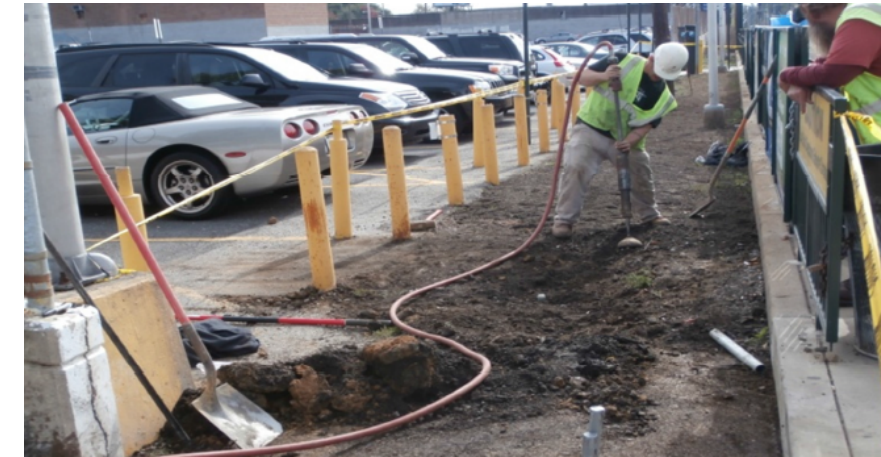
RRD Fox Chase Buried Conduit Installation
