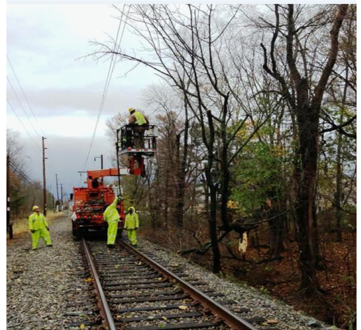
A wire train crew worker heads up to repair Regional Rail catenary.
